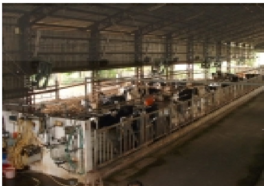
Fig. 1. Shed for dairy cattle equipped with fans. Note the open sides of the shed to promote ventilation
