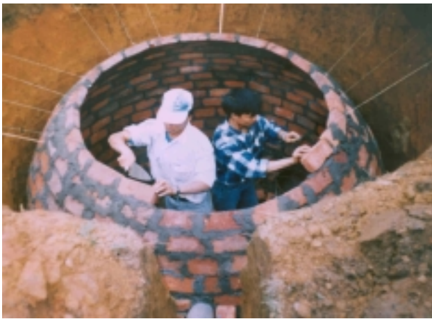
Fig. 3. Building a brick biogas plant with vaulted cover.
