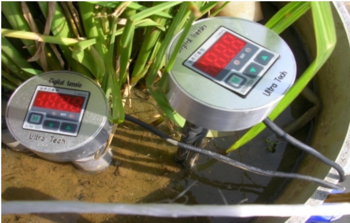
Figure 5. Digitalized submerged water level depth measurement sensors
